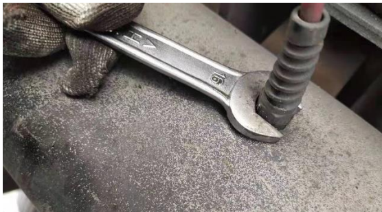
Figure 24: Tightening of waterproof strain relief
