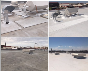
NAVFAC-SW Roofing Project
