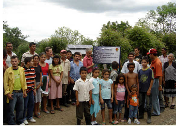
SEI helped Grupo Fenix technicians install a solar electric system on a rural school in Nicaragua
