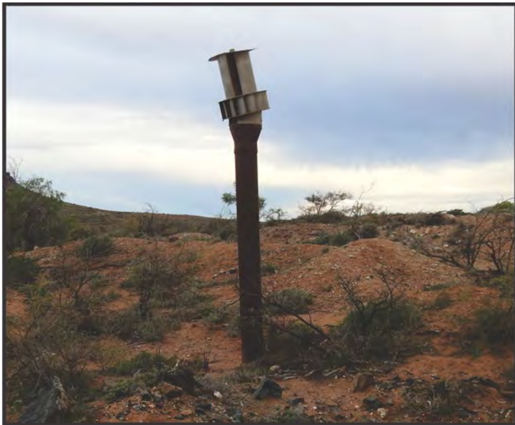
Photo 3-5: Small Vent Shaft Source: ERM
