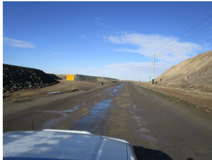
Figure 2: Bunding adjacent haul road
