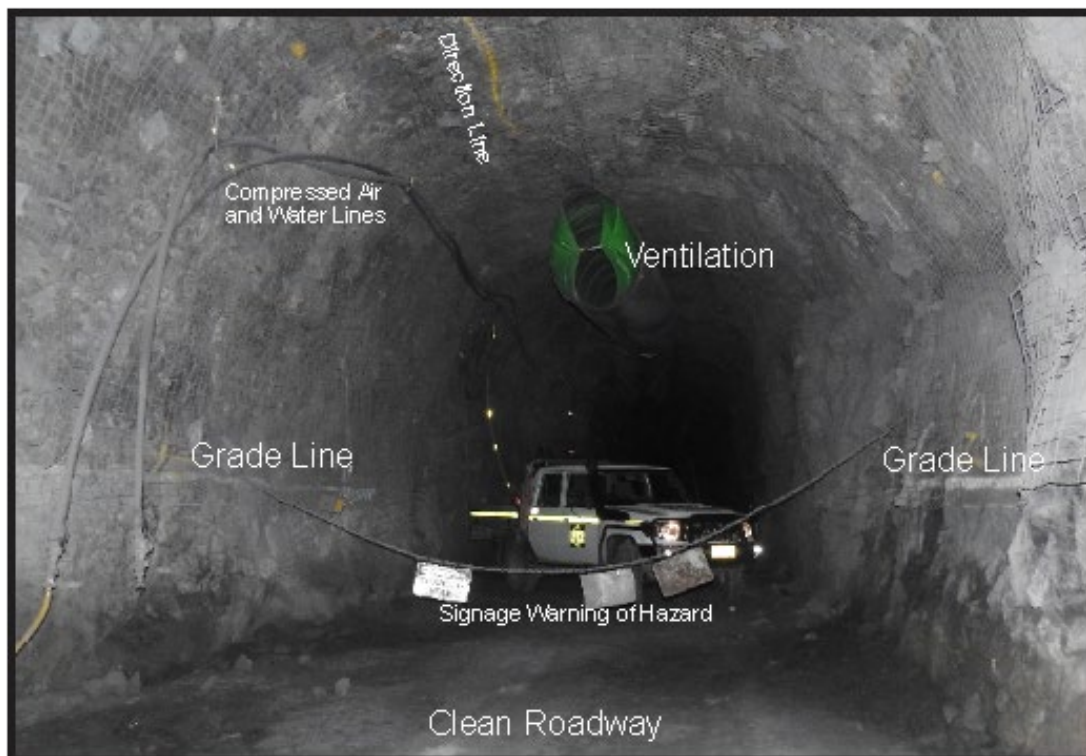
Photo 3-2: Conditions of the Access Roadway Source: ERM
