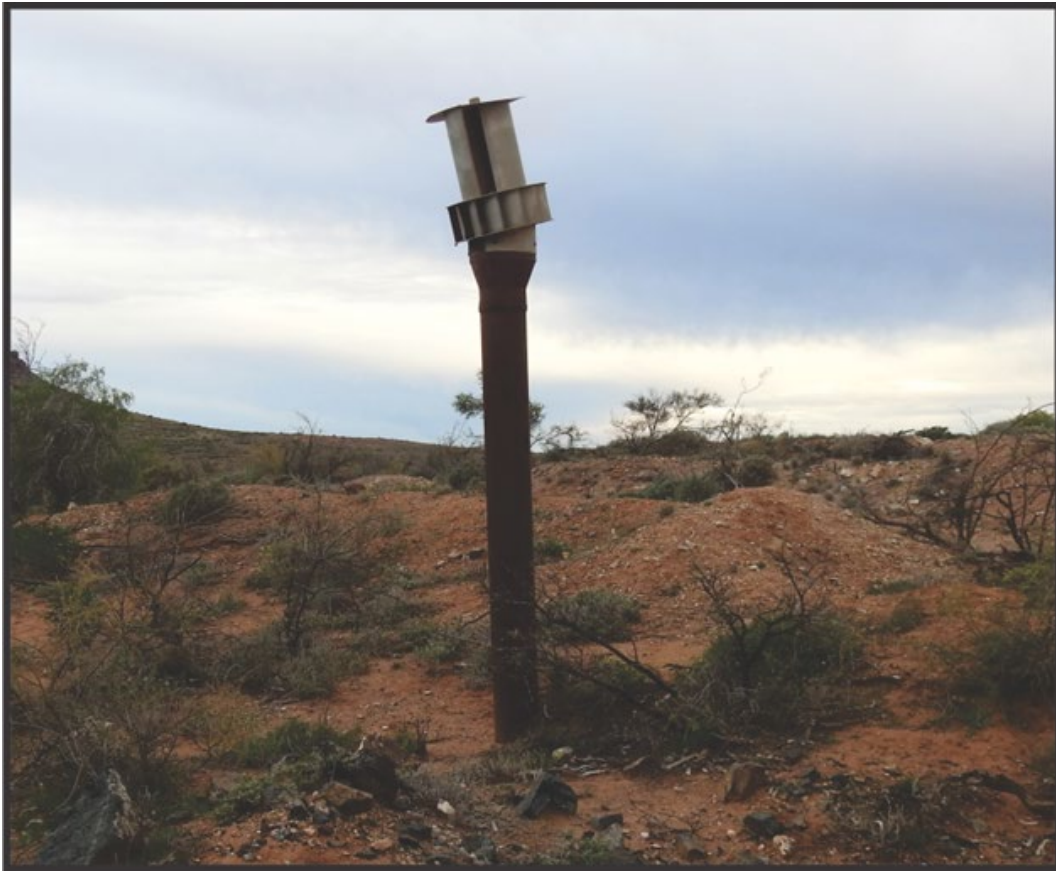
Photo 3-5: Small Vent Shaft Source: ERM
