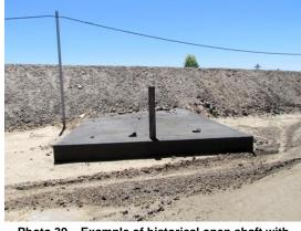
Photo 39 – Example of historical open shaft with concrete cover
