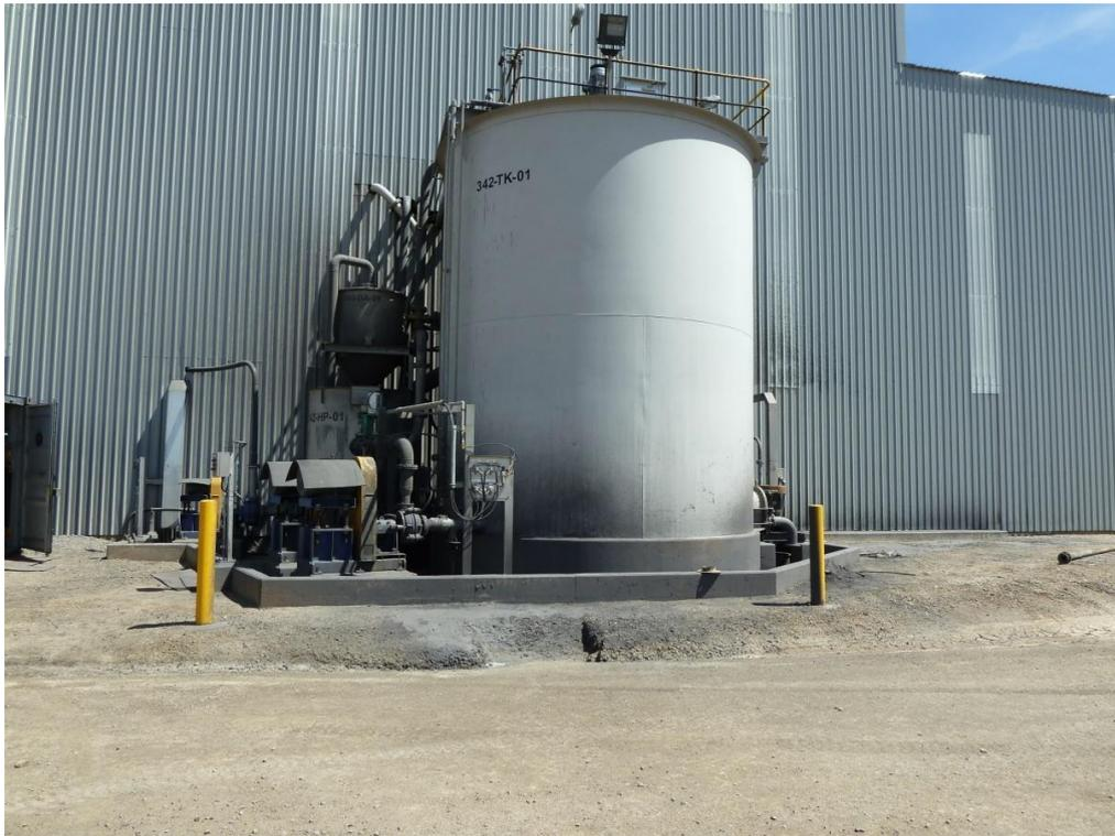
Photo 9. Inadequately banded lead concentrate tank.
