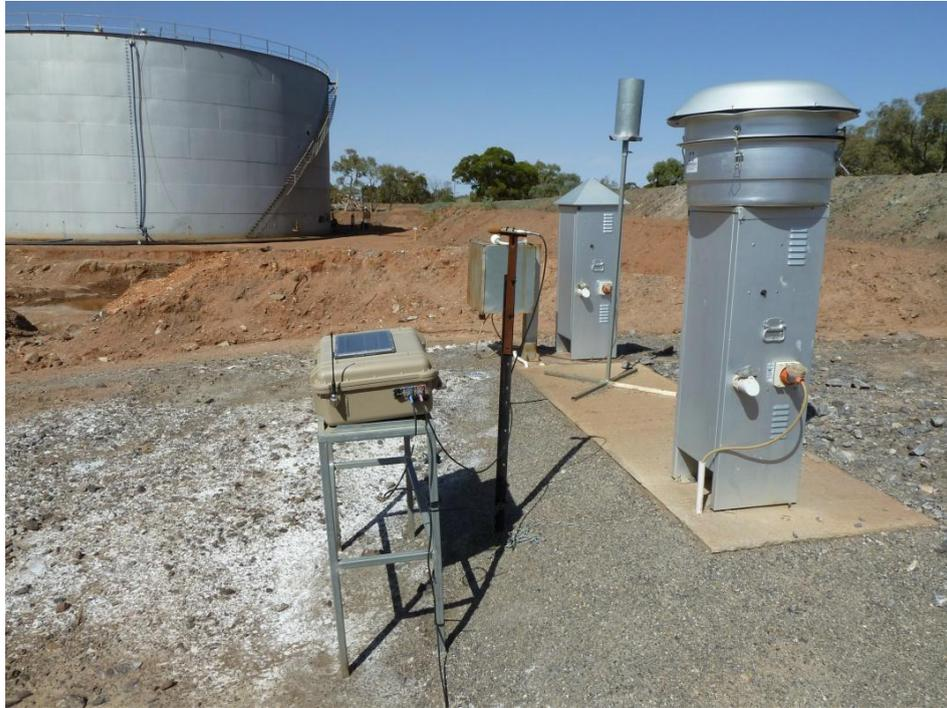
Photo 1. Automatic air monitoring station, noise and vibration monitors.
