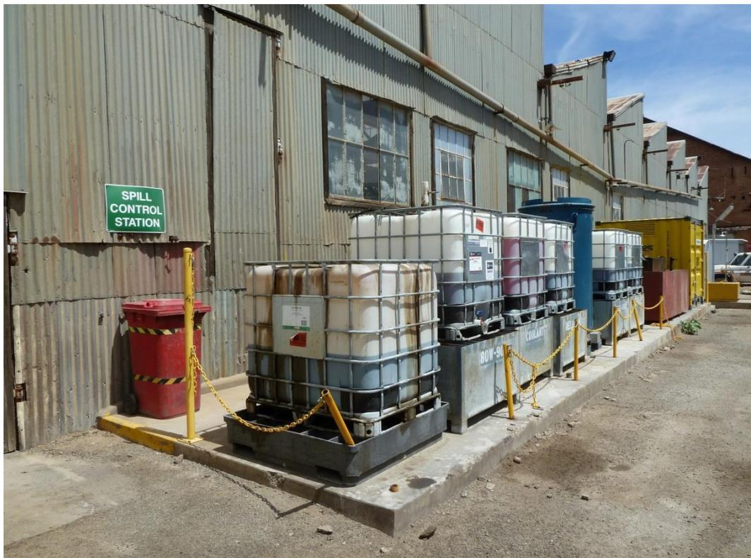
Photo 8. Hydrocarbon storage area with spill kit.
