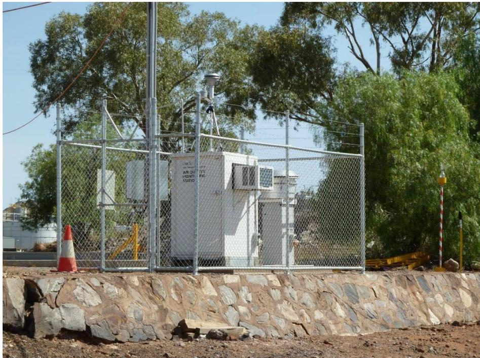
Photo 2. Automatic air quality monitoring station, dust deposition monitor and noise monitor.
