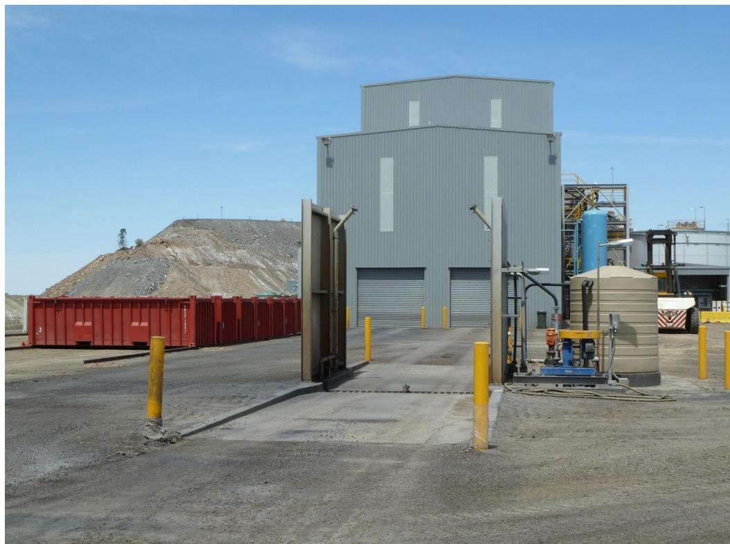
Photo 21. Washdown for trucks and concentrate containers leaving processing plant (in background).
