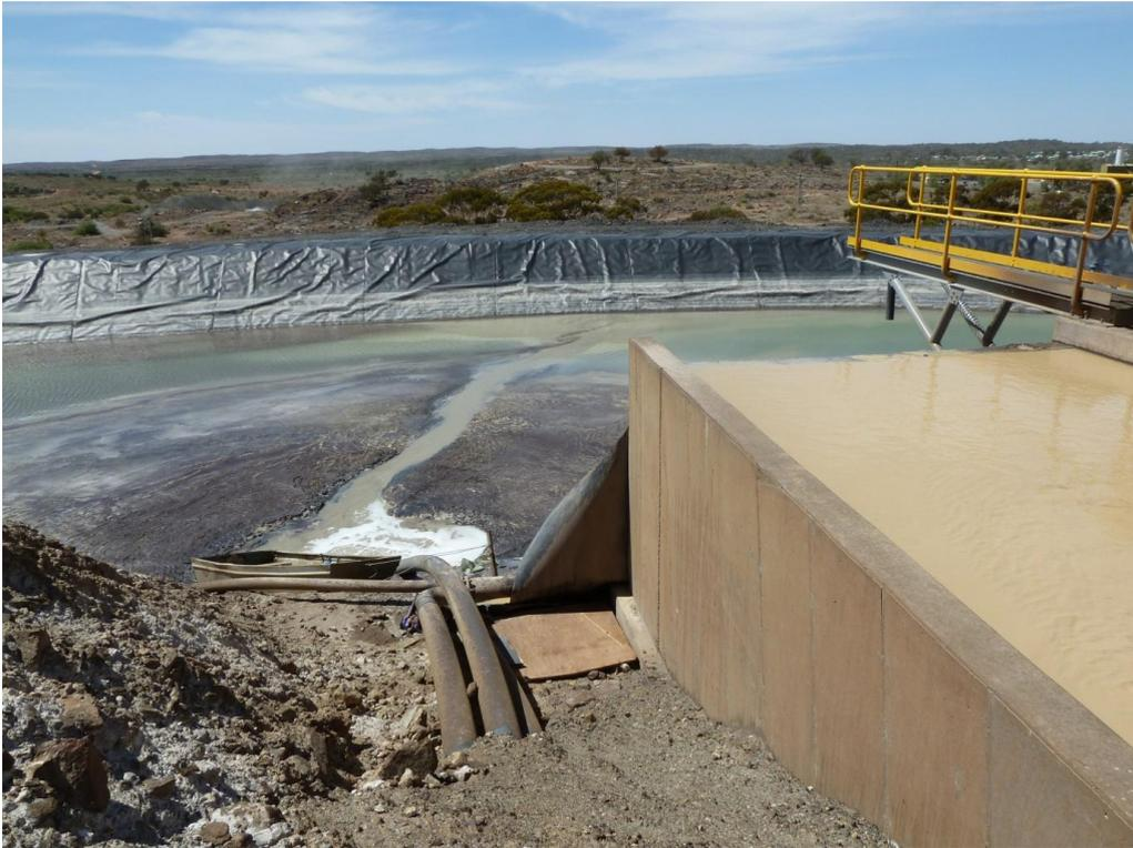
Photo 11. Lined storage pond for water from the water treatment plant.
