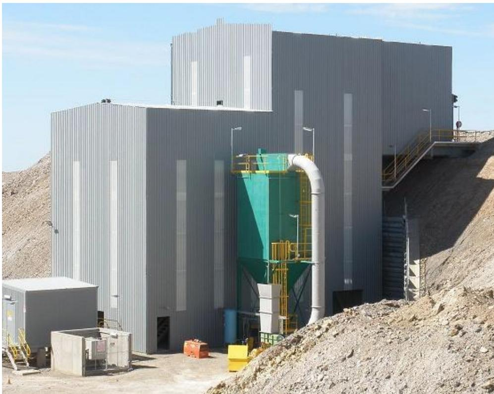
Photo 23. Crusher enclosure and bag house. (Photo by Rasp Mine).
