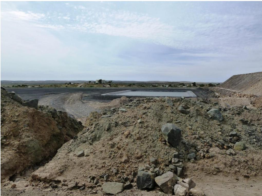
Photo 25. TSF 1 capped with slag and a lined water storage.
