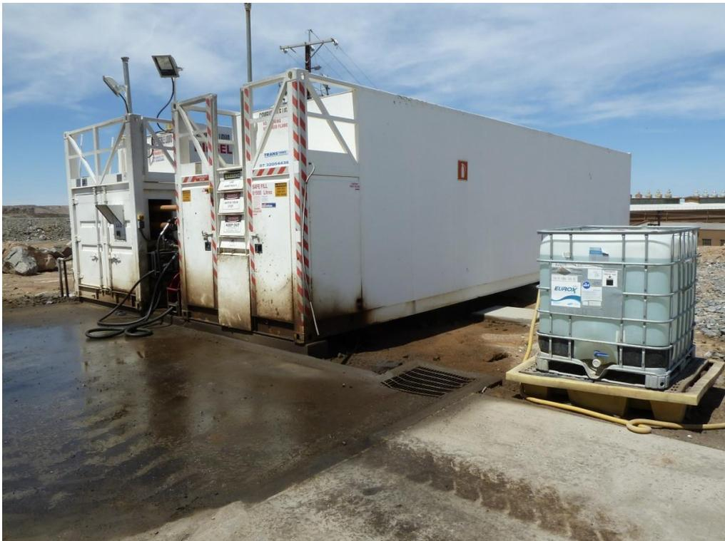
Photo 10. Internally banded 63,000 litre diesel Transtanks. The sump discharges to an oily water separator.
