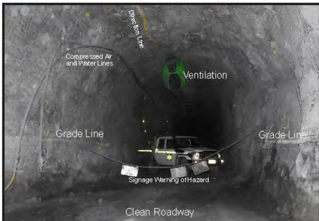
Photo 3-2: Conditions of the Access Roadway Source: ERM
