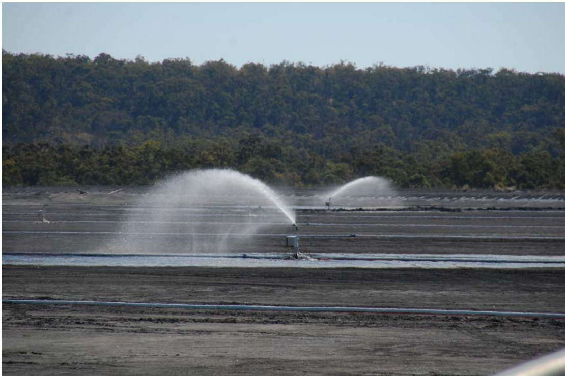
Viva Energy Stack Demolition Dust Suppression
