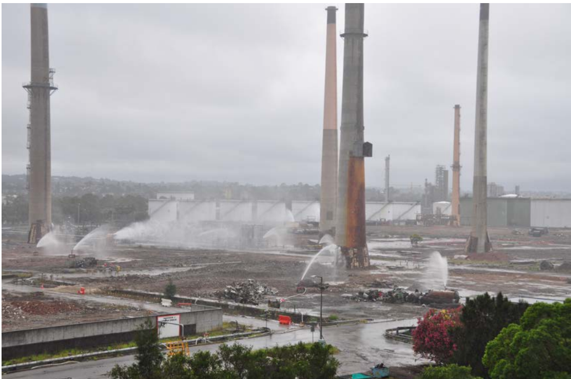
Viva Energy Stack Demolition Dust Suppression
