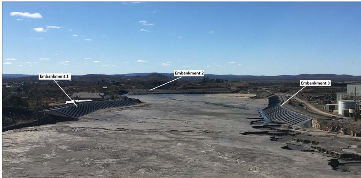
Figure 4-1 View of Embankments 1, 2 and 3
