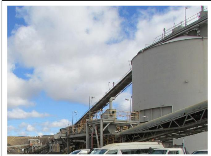
**Photo 23** – Enclosed conveyors from Crusher enclosure to Mill (5 July 2023)
