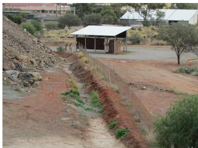
**Photo 6** – TSF2 embankment and trench as cleaned-up after TSF2 embankment seepage incident of 24 December 2022 (5 July 2023)
