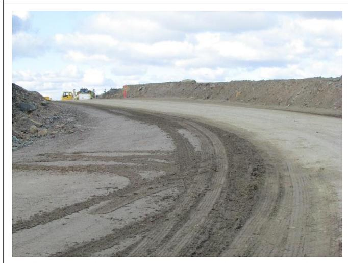
**Photo 21** – Heavy vehicle tyre tracks off sealed road surface on road from rail loadout area to Mill (5 July 2023)
