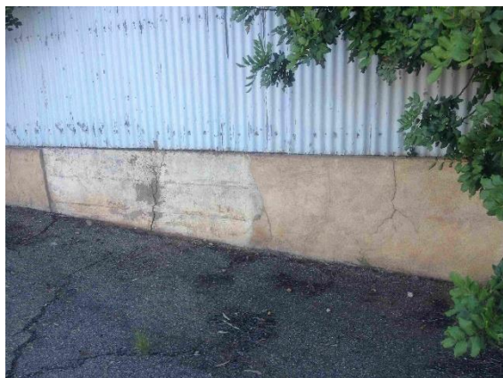
Cracking and deterioration of old concrete fencing and cracking in the asphalt in front of the buildings is evident
