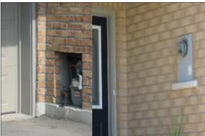
Figure 19: Place hydro and gas meters and other utilities in concealed or recessed locations
