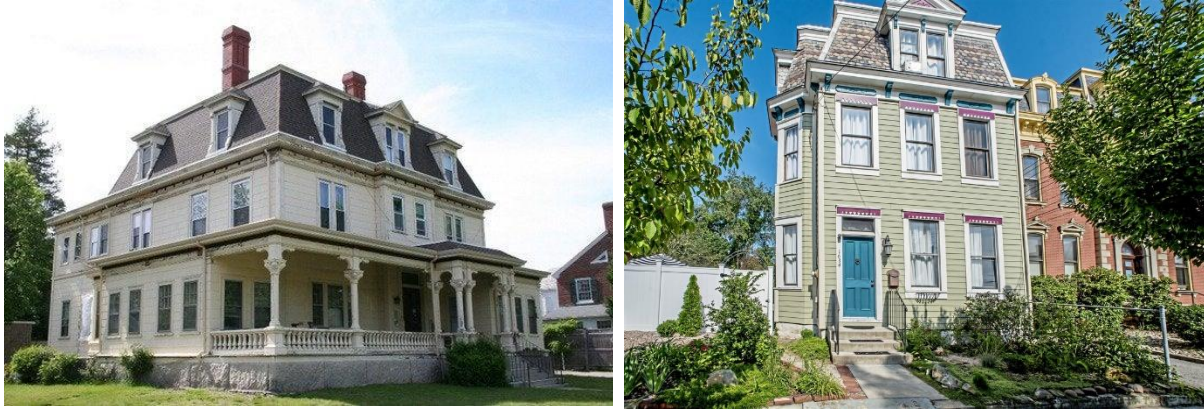
Examples of Traditional 3-Storey Building Designs with 3 rd Floor Incorporated into Roof Design
