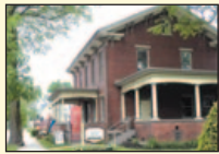
LATTIMER HOUSE 400 W. Mahoning St.
