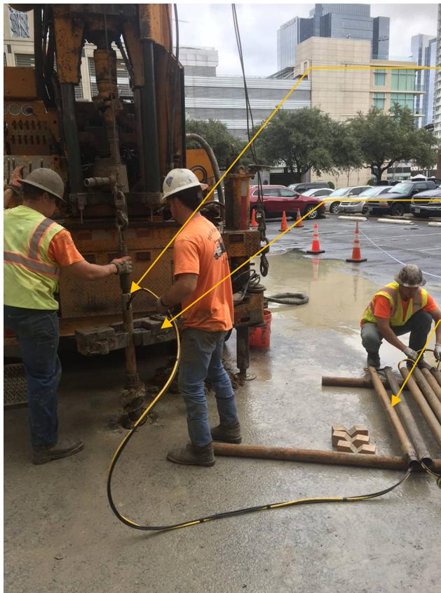
Slotted sub allows the lowering of probe assembly with hydraulic and communication lines protected within core steel/casing.
