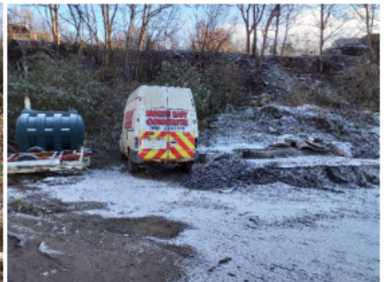
Figure 2.4: Potential landslip and instability of steep slopes in north-eastern section of the site.
