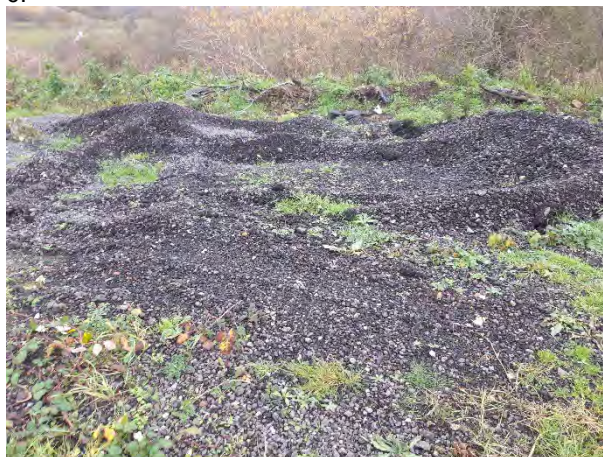
24.11.22 – Poorly spread gravel in northwest corner of site
