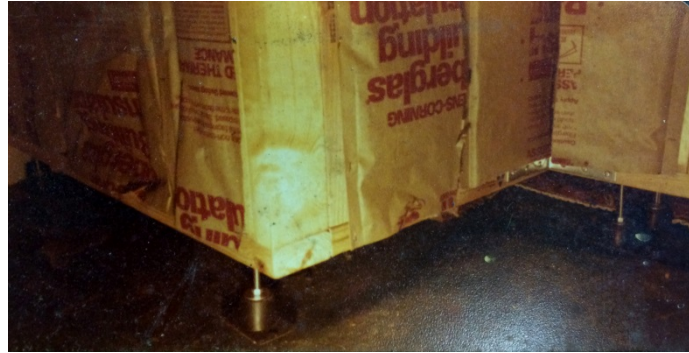
Figure 4. Walls shown floating on neoprene isolators
