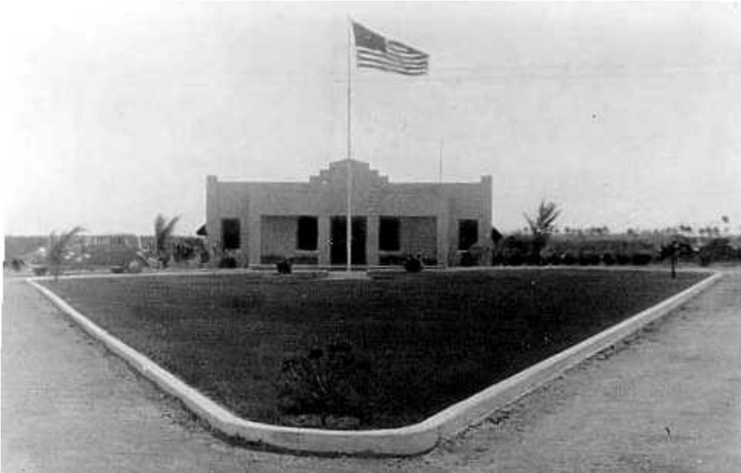
A WW2-era view of Chapman Field's Administration Building
