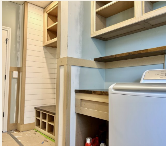
Install in progress
