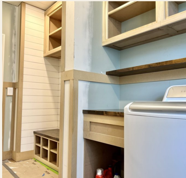
Cabinets and vanity installed, butcher block dry fit
