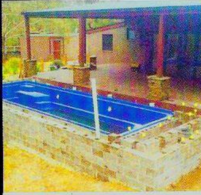
Block Work Around Pool
