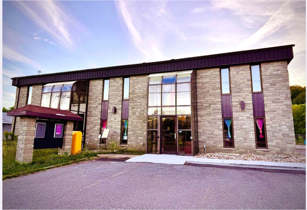
19 Valleyview Drive, Bancroft
