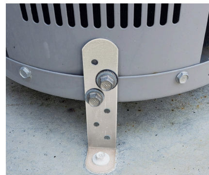
#008-774A 6" CLIPS + 8 SS TEK SCREWS DRILL BIT & SS TAPCONS
