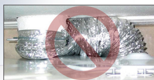
Unprotected Hose is a Fire Hazard
