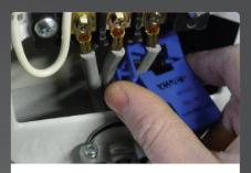
**STEP 3** Disconnect power to clothes dryer & clip current sensor onto a hot conductor in the dryer wiring compartment.
