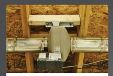
**STEP 1** Mount dryer booster fan and connect to ductwork using the cleanout sleeves.
