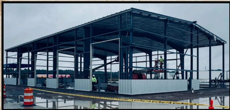
AWG Vehicle Maintenance Facility - Hernando, MS
