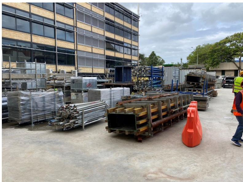
**Figure 3.14: Laydown area for delivery and storage of materials, formwork and scaffolding**
