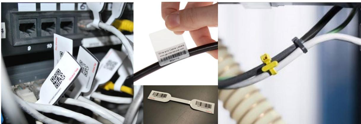
**Figure A8: Examples of cable identification and tracing in buildings** <sup>218, 219, 220</sup>
