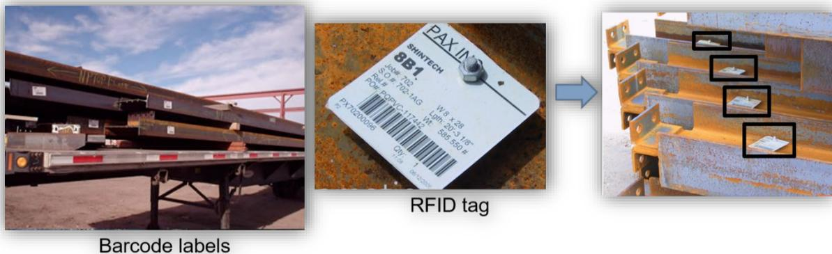
Figure A1: Tracking structural steel using barcode and RFID <sup>204, 205</sup>
