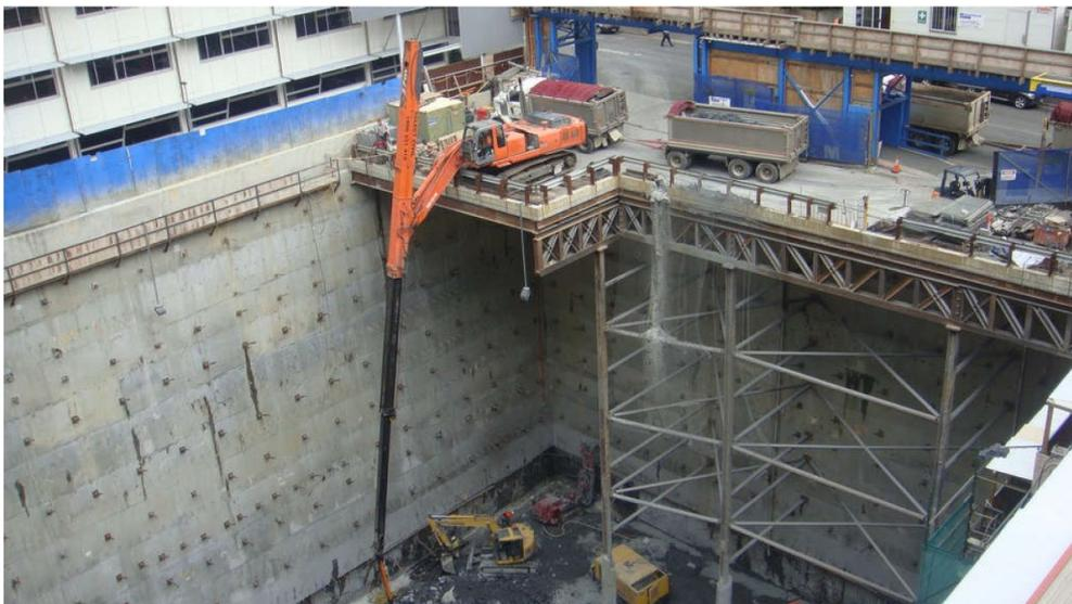
**Figure 3.1: Excavation required before commencing the physical building**
