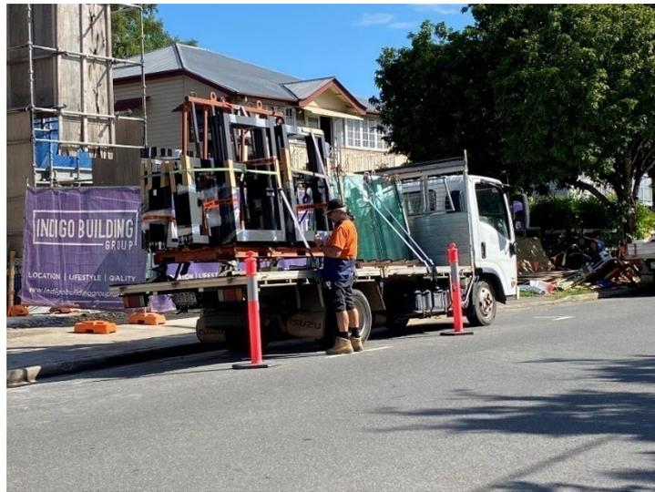
**Figure 3.19: Window frames and glazing being delivered to site**
