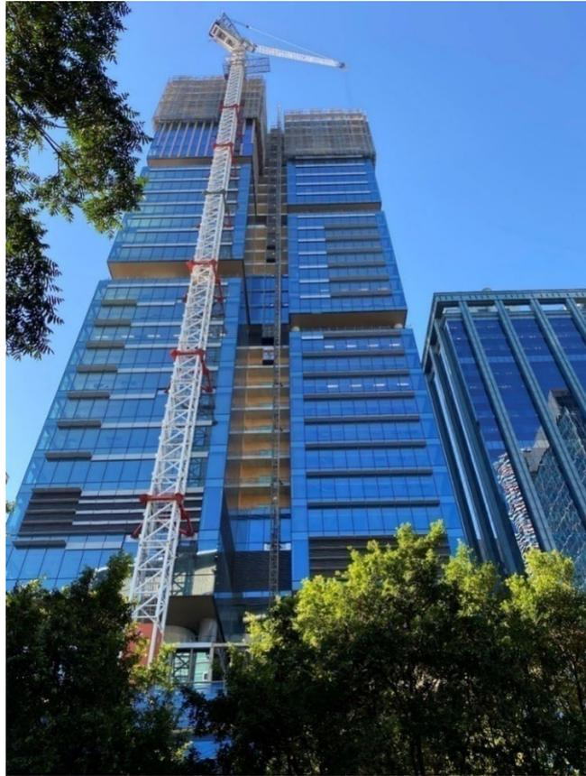
***Figure 3.15: Tower crane and personnel hoist for vertical transportation on multistorey building***
