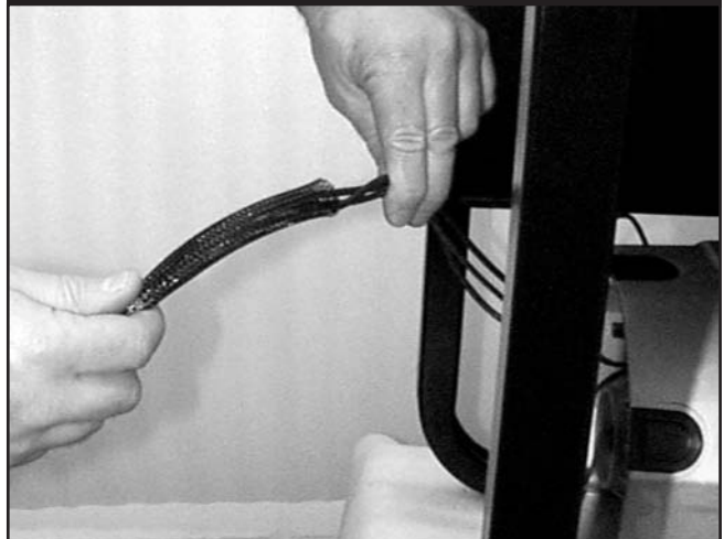
Figure 4.36 — Install Mesh On Cable
