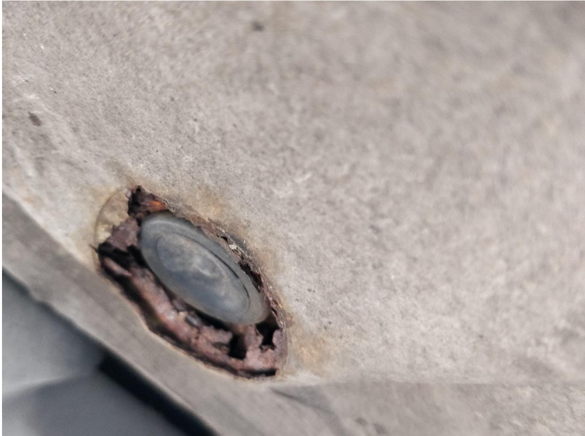
Corrosion
