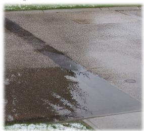
All confirmed that the roadway needs to be appropriately graded to ensure that the water automatically flows from the source(s) to the central drain. That work will commence soon—exact date TBD.
