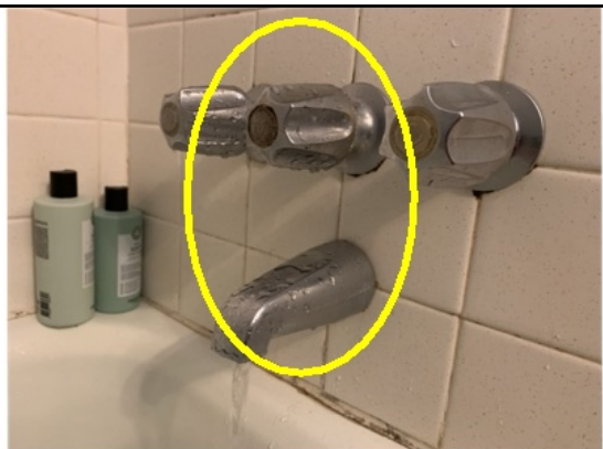
Leaking - master bath
