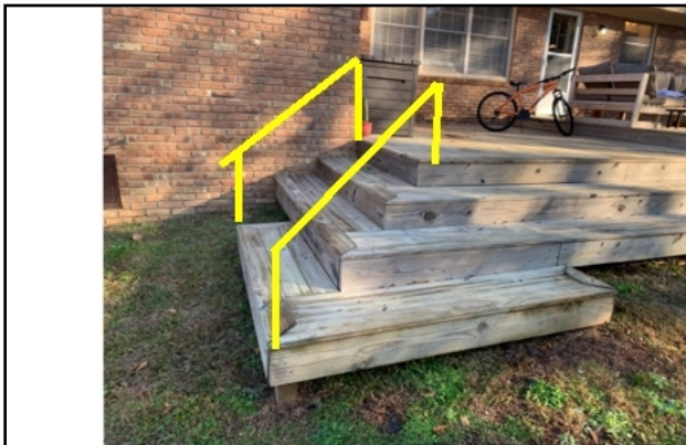
Missing handrails
