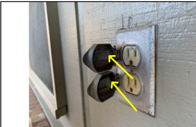
Missing/worn seal
