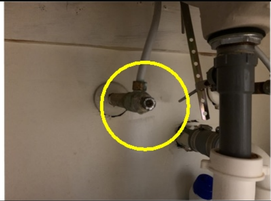
Hallway- shut broken handle
