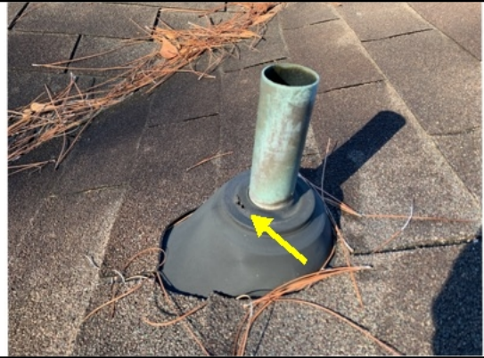
Rubber flashing/boot worn
