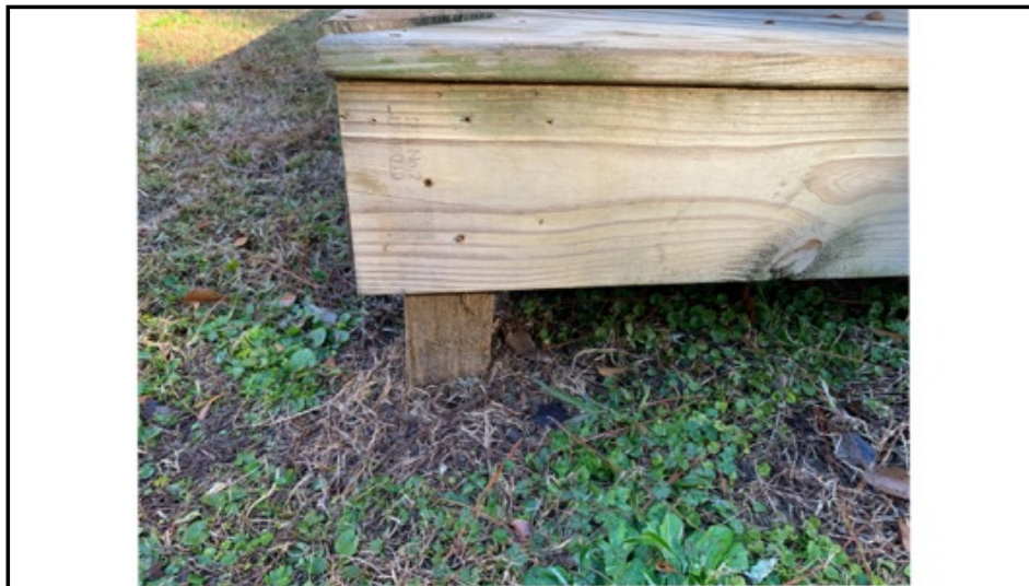
Wood to ground contact
