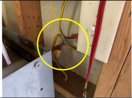
Improper wiring
