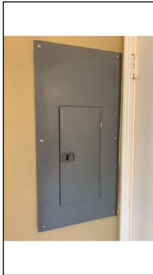
Panel screws stripped
