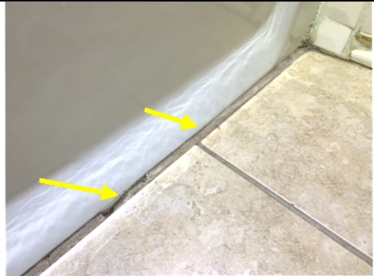
Hallway- tub/floor needs sealing
