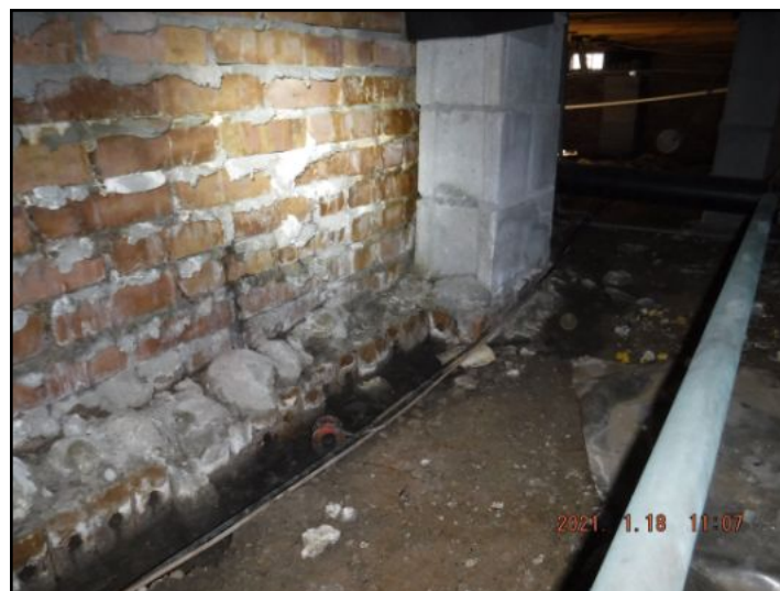
Moisture along exterior wall
