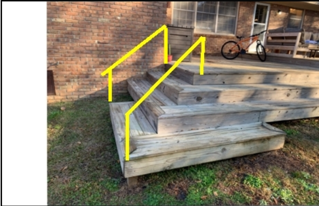
Missing handrails
