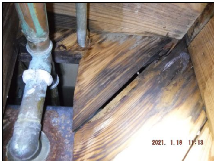
Moisture damaged/elevated moisture - bathroom area
