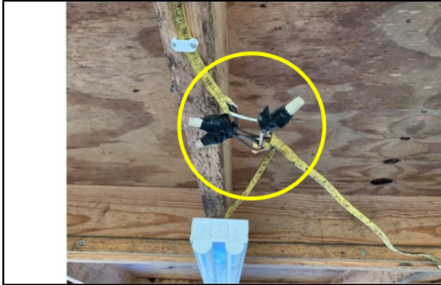
Improper wiring
