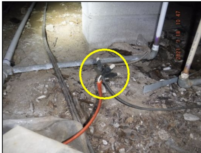
Improper electrical connection
