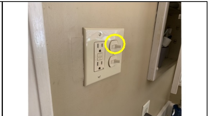
Top switch does not operate
