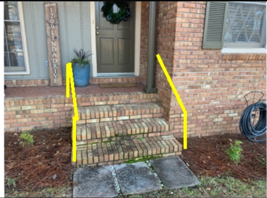
Missing handrails
