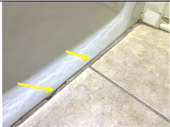
Hallway- tub/floor needs sealing
