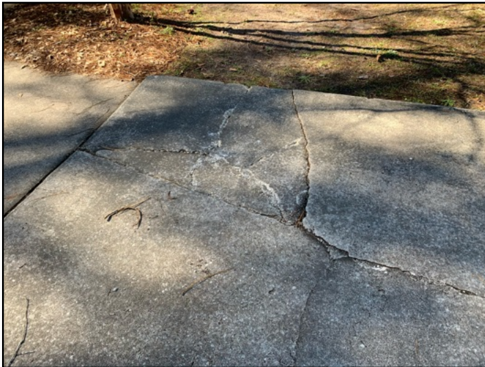
Driveway cracks
