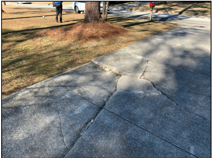
Driveway cracks
