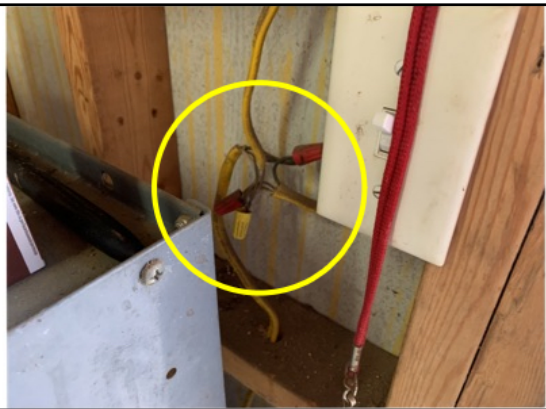
Improper wiring
