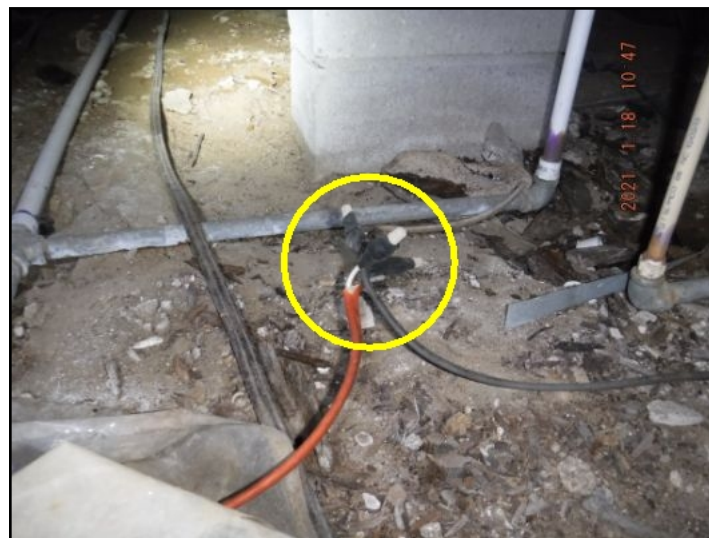
Improper electrical connection
