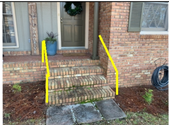
Missing handrails
