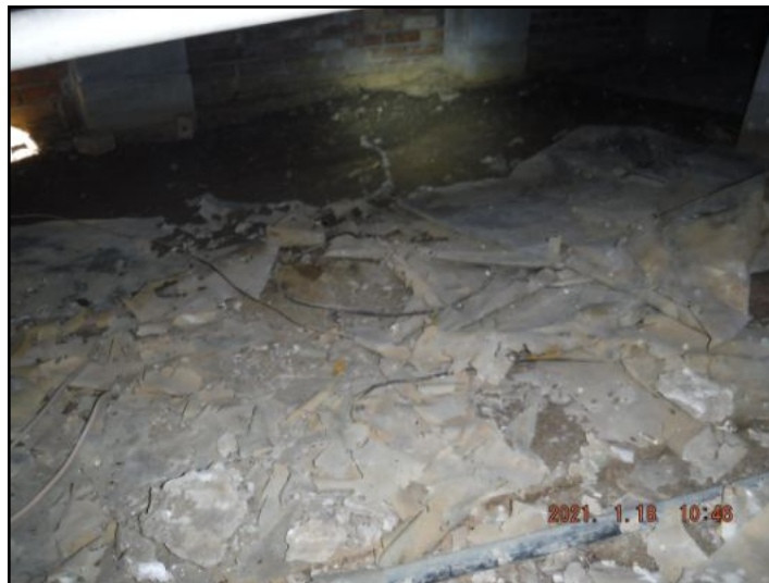
Vapor barrier in disrepair
