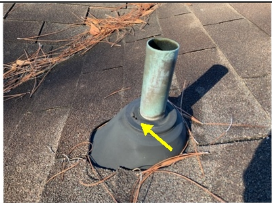
Rubber flashing/boot worn
