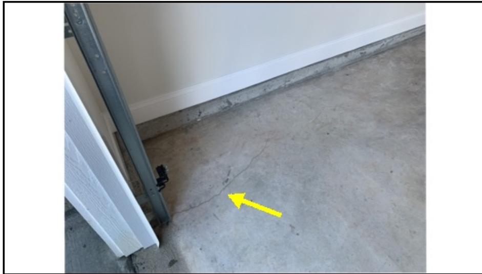
Typical settlement crack
