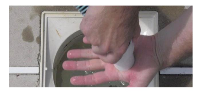
If a vac plate is being used, attach it to the end of the hose that was up against the return jet, block the opening, and bring it over to the skimmer. Be sure to create a good seal or suction will be lost.
