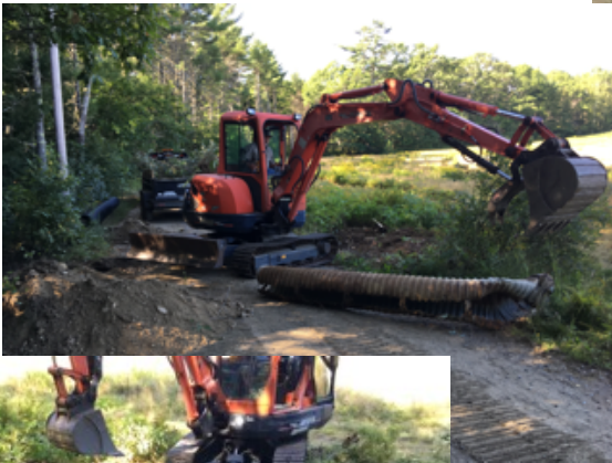
Below: Culvert work from 319 Grant
