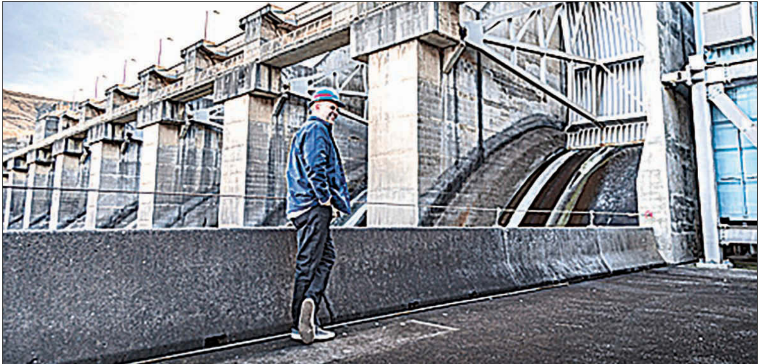
Social media content creator Adam Ratliff, the "Armchair Engineer," takes a tour of Lower Granite Dam. Ratliff is working on behalf of the farmer non-profit Center for Sustainability and Working Rivers to educate the public about the benefits of the lower Snake River dams. (Courtesy Adam Ratliff)
