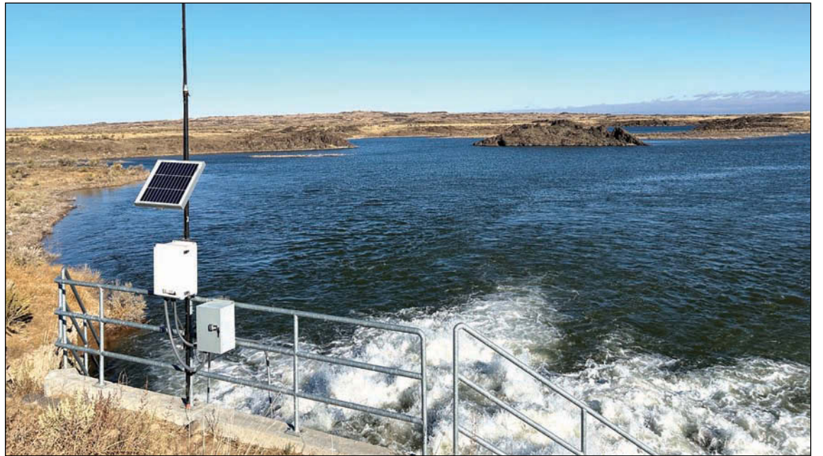
Milepost 29 aquifer recharge basin in southern Idaho. (Courtesy Idaho Department of Water Resources)
