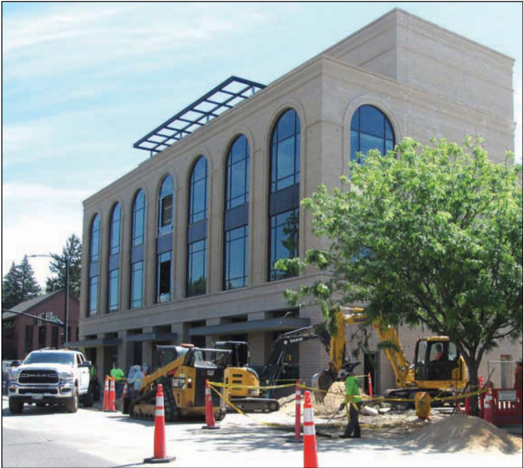
Idaho Wheat Commission building construction June 24, 2026, in downtown Boise. The commission expects to move into the multi-tenant building in August. (Brad Carlson/Capital Press)
