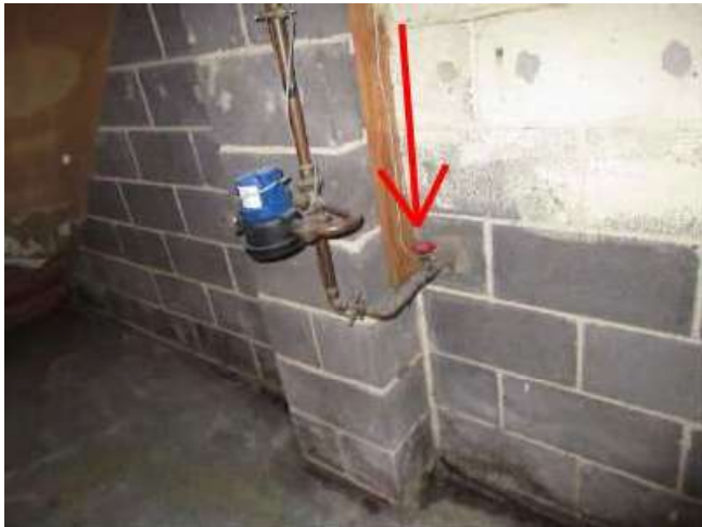
Photo X-4 Main Water shut off
