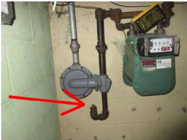
Photo X-2 Main Gas shut off
