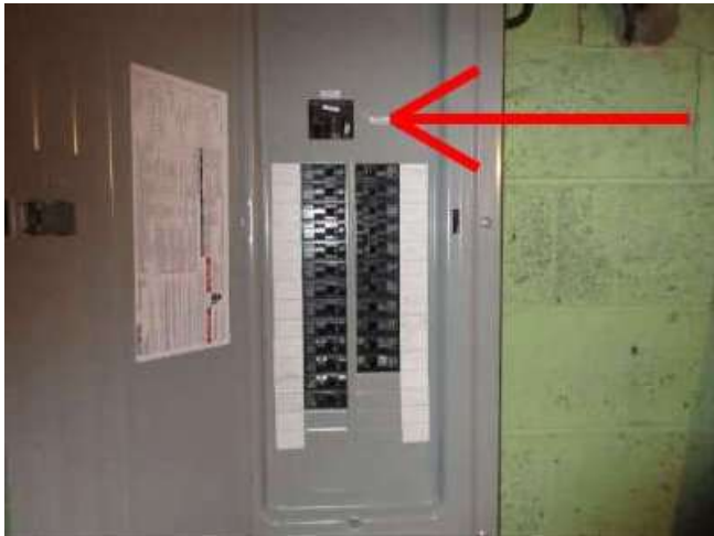
Photo X-3 Main Electric shut off
