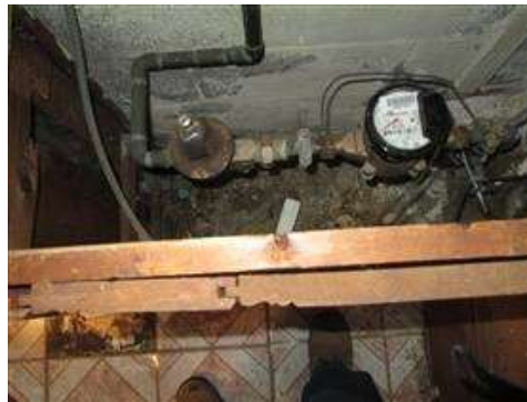
Photo X-2 Water meter and main water shutoff
