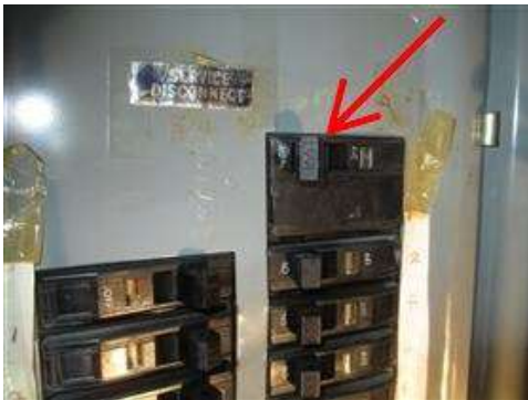
Photo X-1 Main electric shutoff
