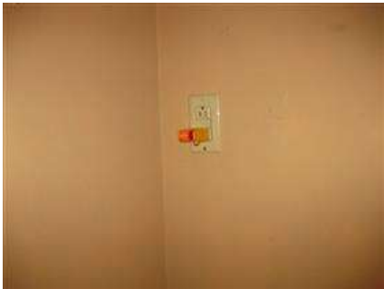
Photo 82 2nd floor bathroom
