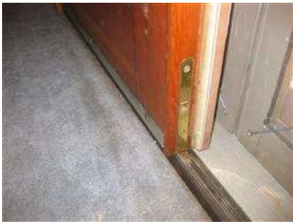
Photo 43 Pin on bottom of double door.
