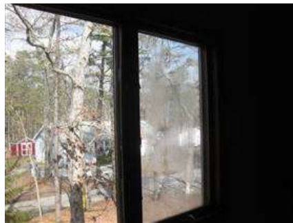
Photo 80 2nd floor north bedroom
