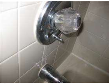
Photo 77 1st floor full bath
