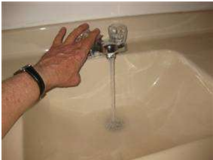
Photo 78 1st floor full bath
