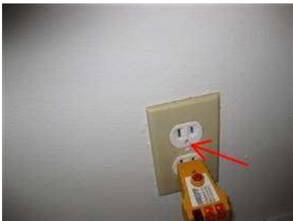
Photo 67 Front North Bedroom
