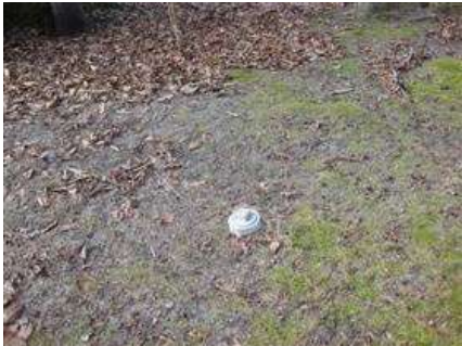
Photo 22 Sewer clean-out in back yard
