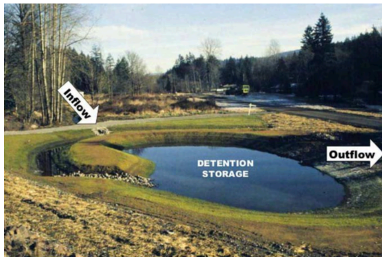
Figure L : Above Ground detention basins Source: Booth & Bledsoe, 2009
