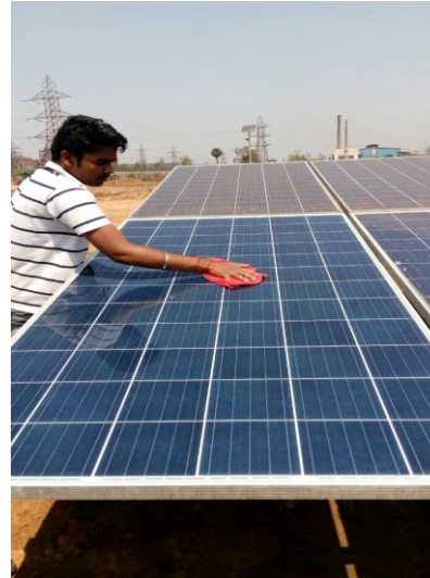
Coating “Solar Glass Shield” solution on Panels.
