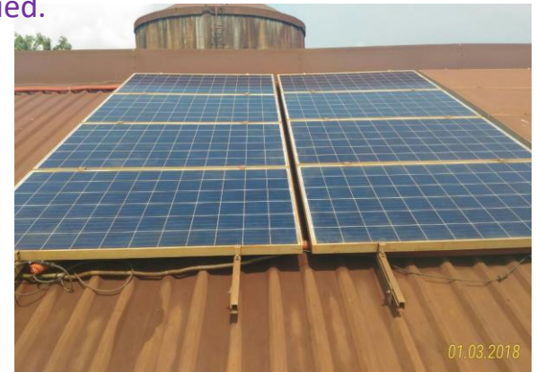
Panels coated with "solar Glass Shield".
