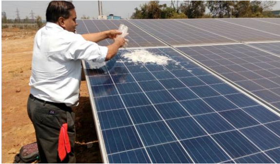
Initial Cleaning with “Solar Glass Cleaning Compound”
