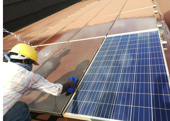
Few Panels of one String cleaned and then "Solar Glass Shield" applied.
