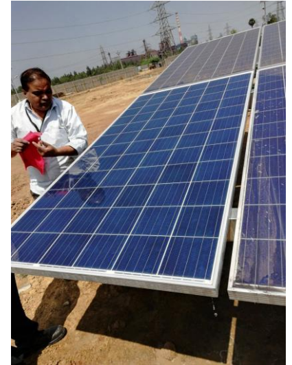
New like finish to the Panel glass after the cleaning and coating application process is complete.
