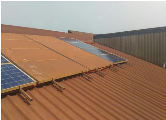
Either side rows coated with "Solar Glass Shield", non-coated in between
