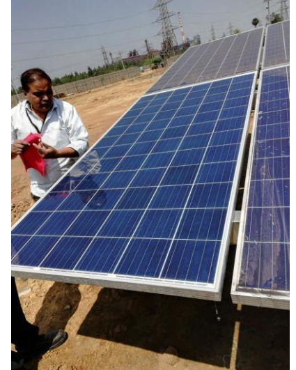
New like finish to the Panel glass after the cleaning and coating application process is complete.
