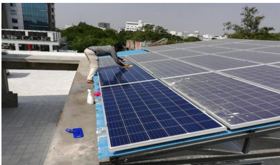
Cleaning with Pre-Cleaner Liquid.
