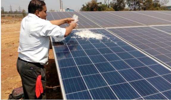
Initial Cleaning with “Solar Glass Cleaning Compound”
