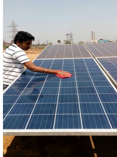
Coating “Solar Glass Shield” solution on Panels.
