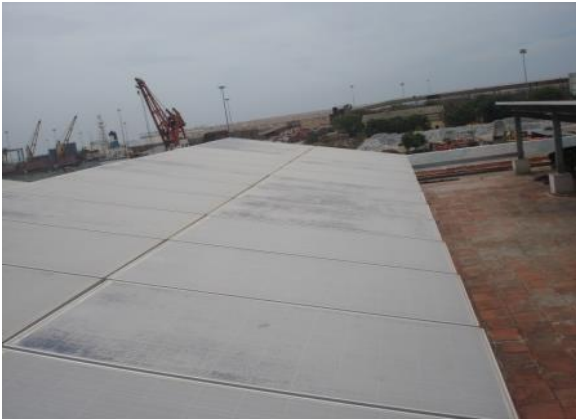
Panel covered with Salt layer.
