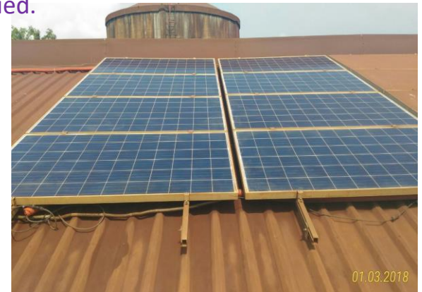
Panels coated with "solar Glass Shield".
