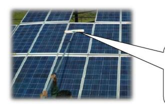
Simple Method of cleaning using Washer with Microfiber Sleeve and Water
