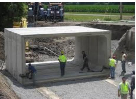
Design flexibility: The box culvert concept has been modified over the years to solve many job-site problems. Standard rectangular boxes are produced in many combinations of height and width. They are approved by Building Code Standards ASTM C1577 provides a table for sizes ranging from 3 ft wide by 2 ft high to 12 ft wide by 12 ft high.
