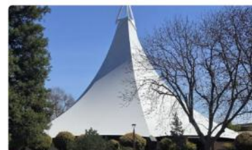
Support New HVAC at Good Shepherd Fresno
