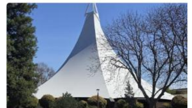
Support New HVAC at Good Shepherd Fresno
