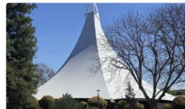
Support New HVAC at Good Shepherd Fresno
